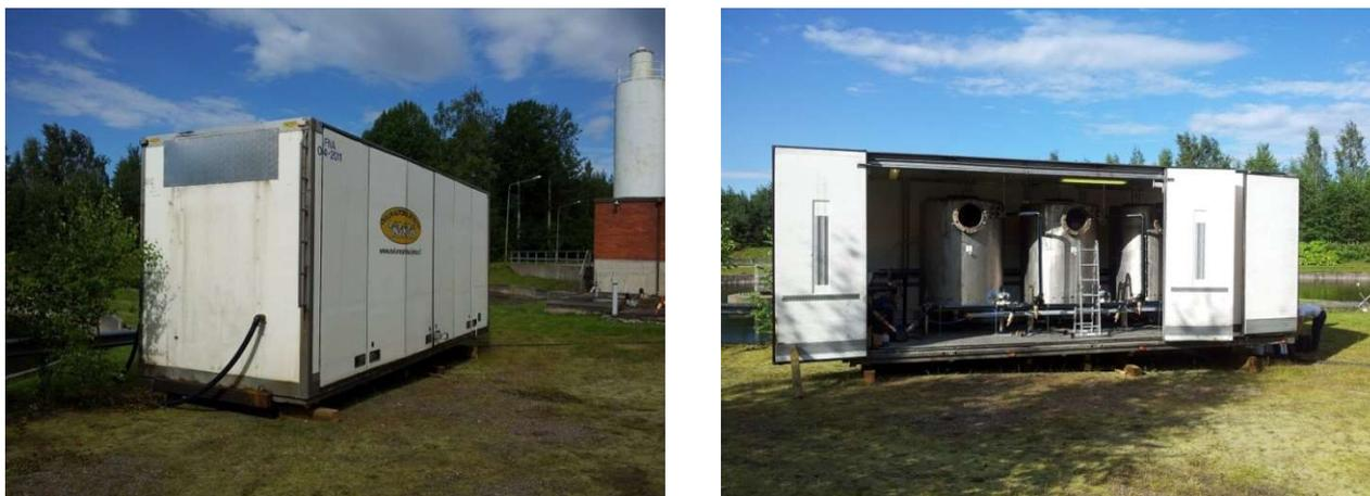
**Figure 2.** a) The filter container from outside and b) filters inside the container.
